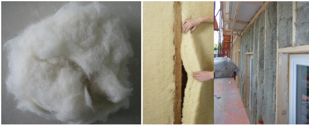
Fig. 1. Photo of sheep wool and its applications in building construction.
